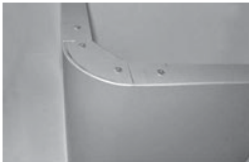
Corner Panel with Gusset & Filler Plate
