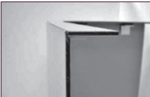
Cope at Edge of Panel
